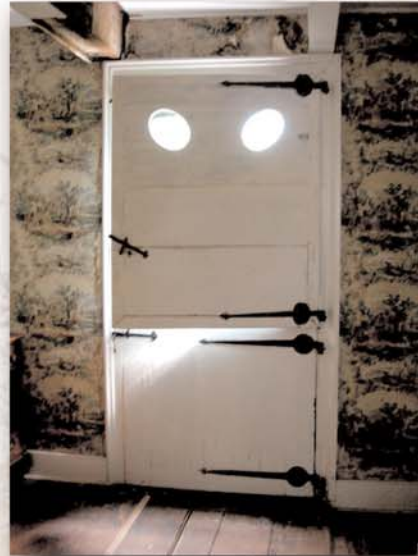
The front entrance Dutch door features distinctive “bullseye” glass panels and original hardware.
